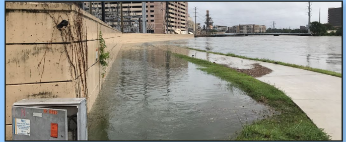
Substation floodwall during Hurricane Harvey.
